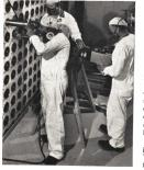
Technicians prepare to remove radioactive samples from face of reactor.
