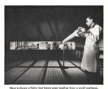
Here is snown a triuty-tool beam pipe leading from a small eighteeninch cyclotron which produces three mev protons. The protons strike a metal target to produce an intense beam of neutrons. Of course no person is permitted in this area when the apparatus is in operation.
